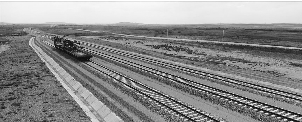
Figure 4. Construction of the railway that stretches to the Zangezur Corridor
