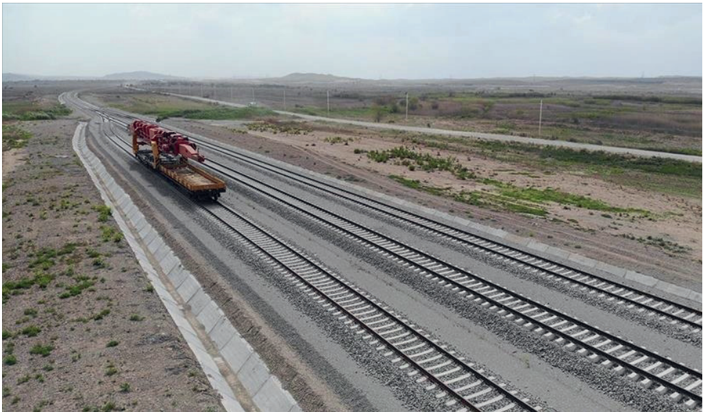
Figure 4 Construction of the railway that stretches to the Zangezur Corridor
